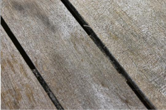
When the timber is fully dry a light sand is required to remove splinters and create a good surface to paint on to.
